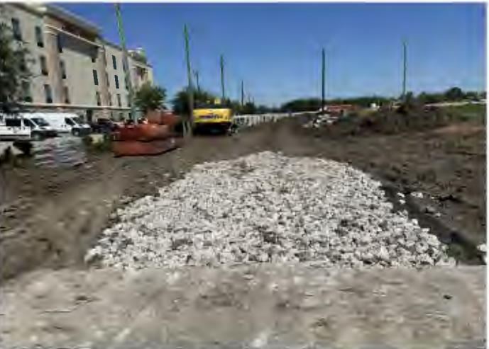
Stabilized Construction Access Installation
