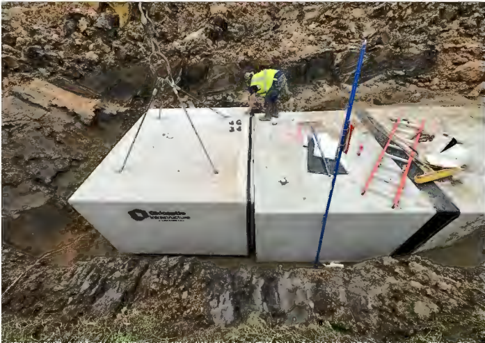
Reinforced Concrete Box Installation
