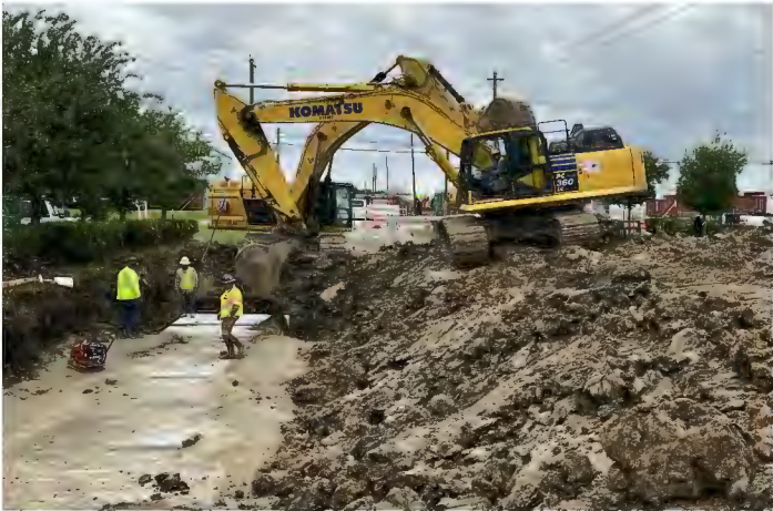
Reinforced Concrete Box Installation
