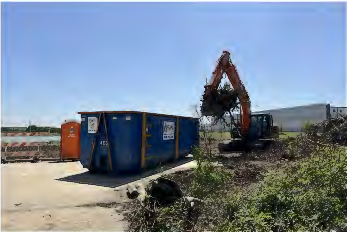
Clearing and Grubbing
