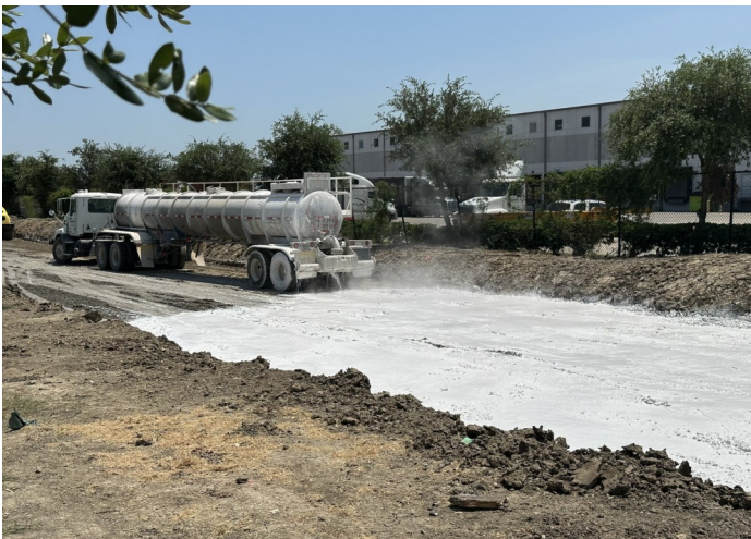
Applying Lime Slurry
