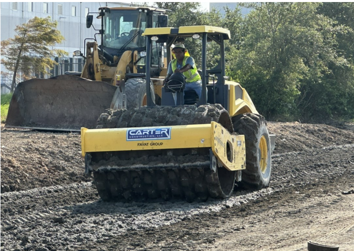
Lime Stabilized Subgrade Mixing and Manipulation
