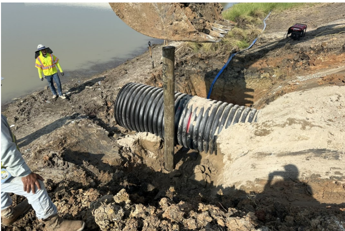
48" Outfall Installation
