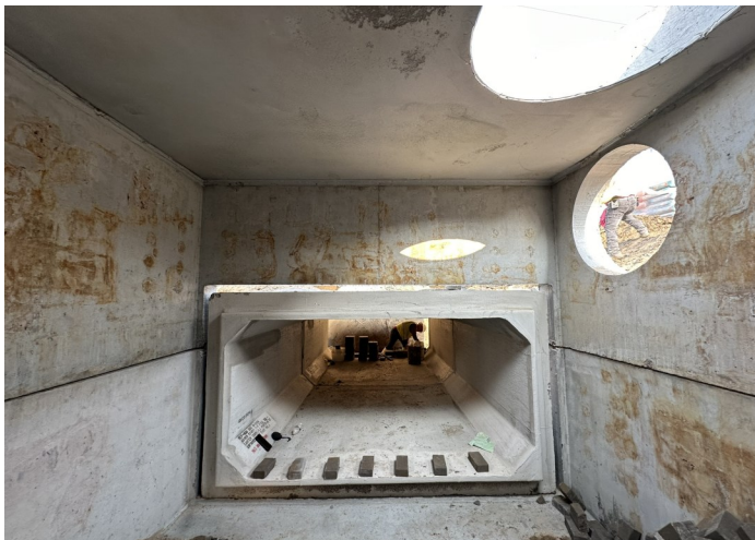
Junction Box and Brick Plug Installation
