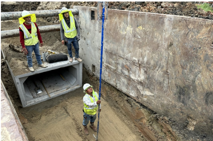
Reinforced Concrete Box Installation
