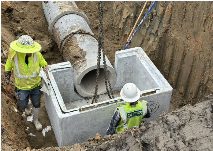
Inlet and Inlet Lead Installation
