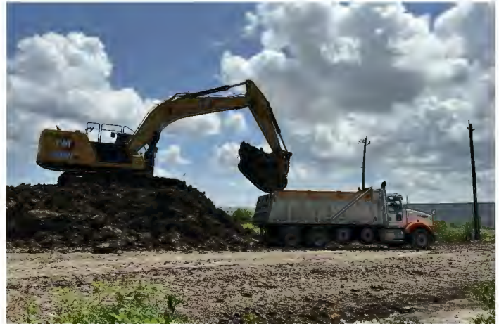
Hauling and Disposing of Soil Offsite
