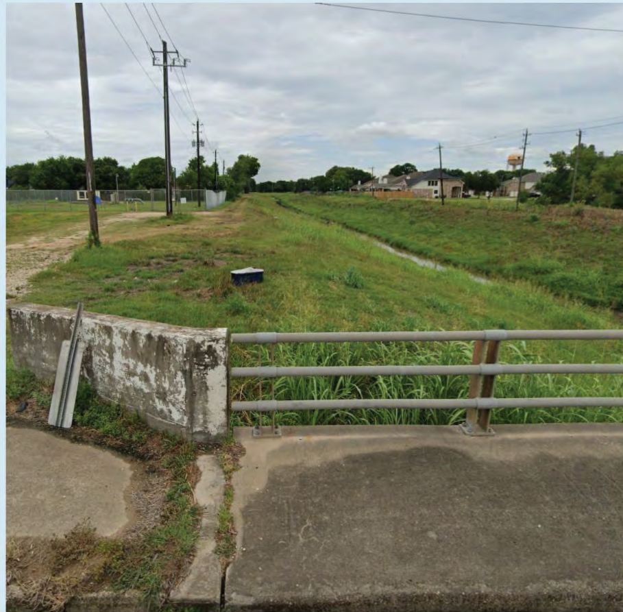
W. FAIRMONT PARKWAY BRIDGE
