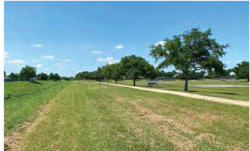
EAST SIDE (NORTH OF SPENCER HIGHWAY LOOKING NORTH)
