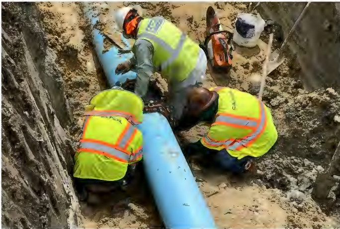
Wet Connection Installation
